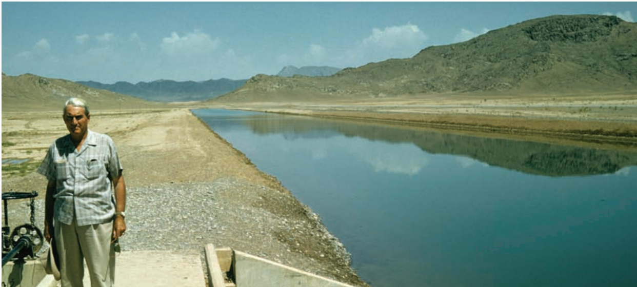
Figure 6. Top: Canals built through Point 4 funding in 1957, courtesy of Boise State Digital Collections. Bottom: Still taken from Arizona and Its Natural Resources , courtesy National Archives.
