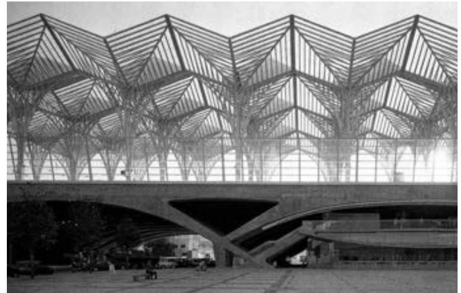
Santiago Calatrava East Station Lisbon, Portugal (1993–1998)
